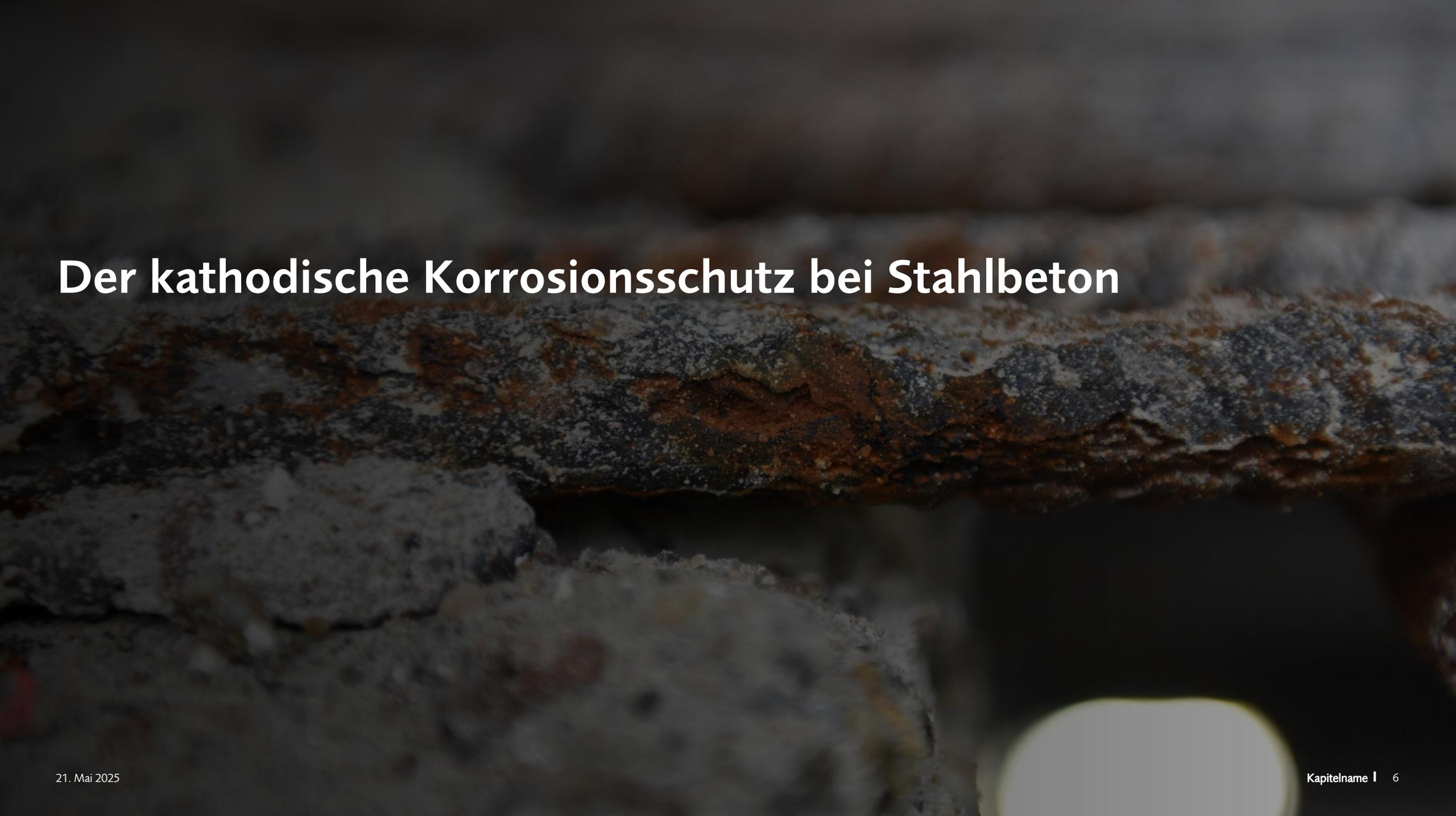
A close-up photograph of a steel reinforcement bar (rebar) embedded in concrete. The rebar is heavily corroded, showing a thick, dark brown and black rust layer. The concrete surrounding the rebar is cracked and appears to be spalling, indicating significant structural damage due to corrosion. The background is dark and out of focus.
